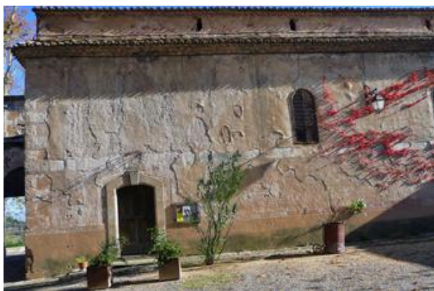
Building before renovation
